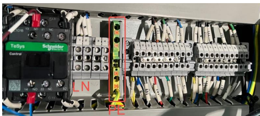
Explosion-proof cabinet power cord wiring position
